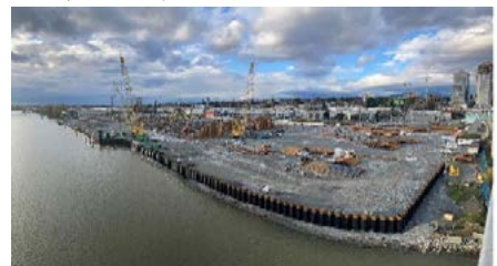
Marpole Transit Centre construction
