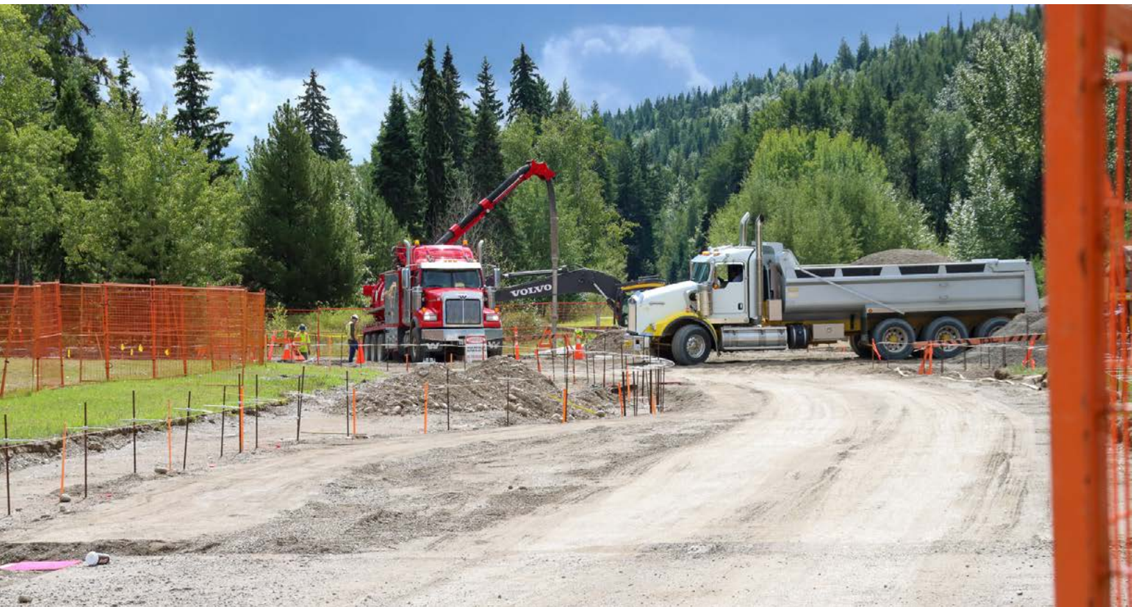
Roundabout under construction in Prince George
