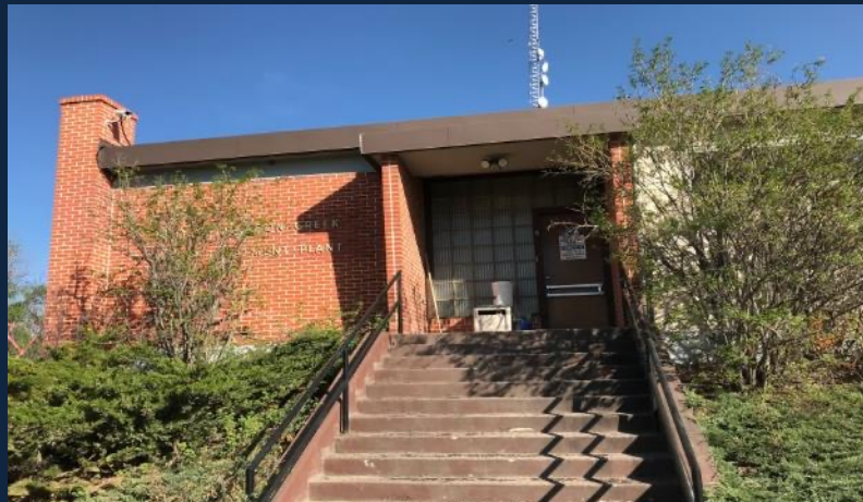
Water Plant & Distribution System
