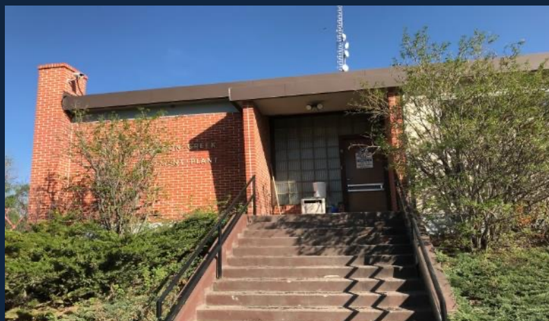
Water Plant & Distribution System
