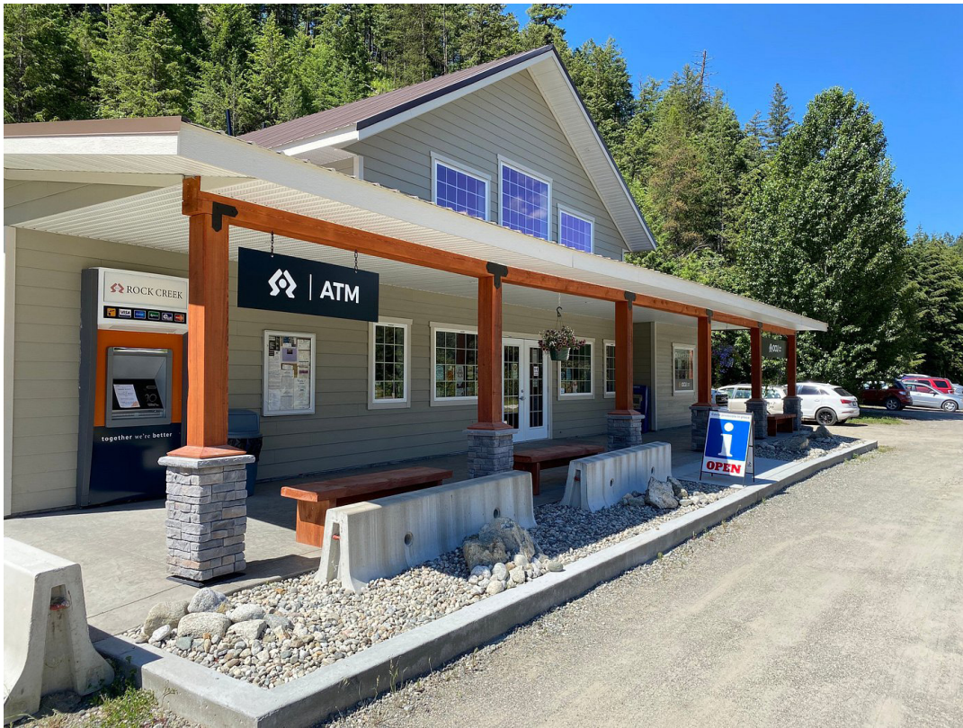
Regional District of Kootenay Boundary / Community of Rock Creek Visitor Information Centre Development
