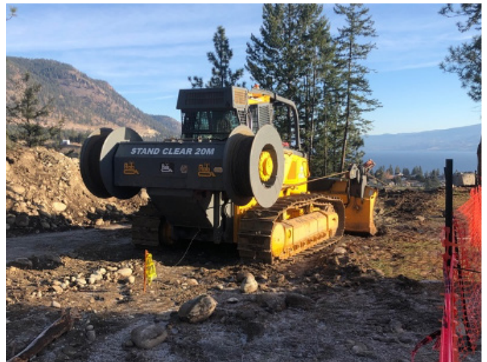
District of Peachland / Trepanier Creek Interconnect
