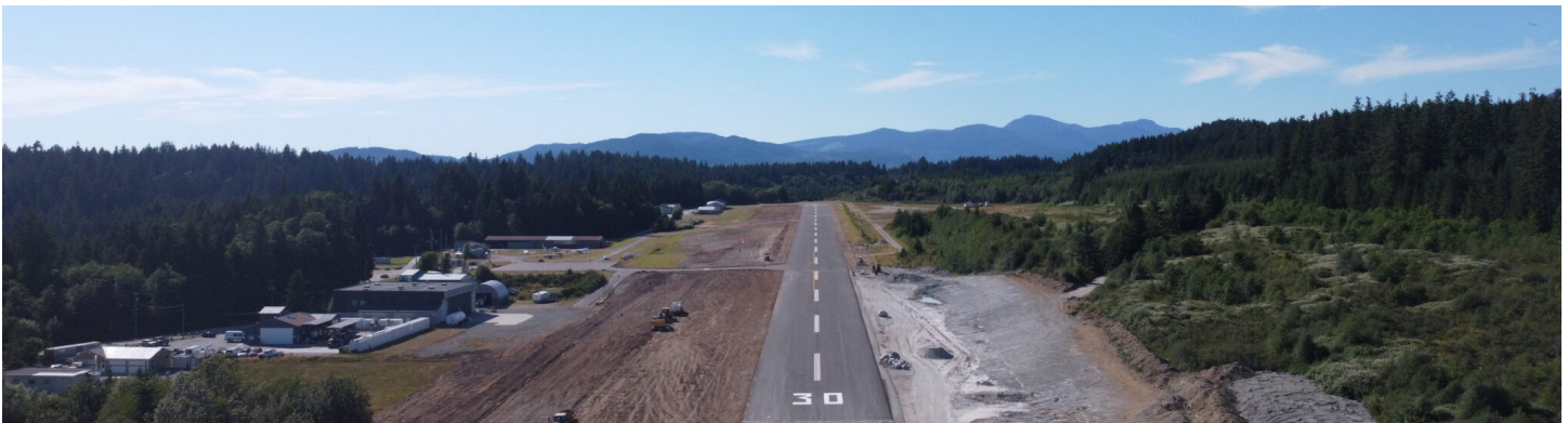
District of Sechelt / Sechelt Airport Runway Lighting Upgrade
