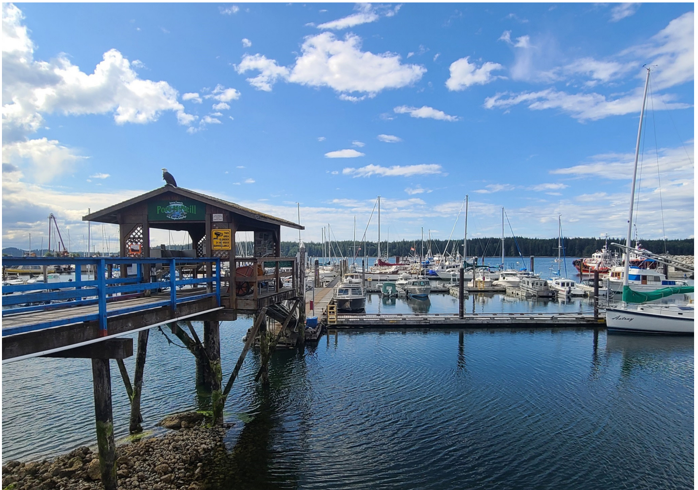
Town of Port McNeill / Municipal Dock and Ramp Replacement
