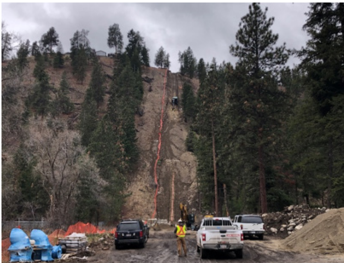
District of Peachland / Trepanier Creek Interconnect
