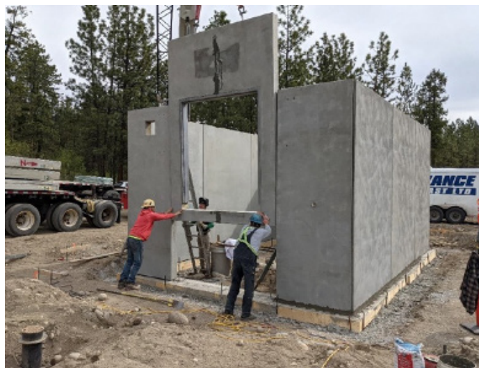
District of Peachland / Trepanier Creek Interconnect
