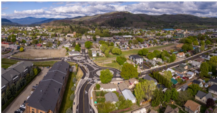
City of Vernon / Double Roundabout at 39th Ave and the 29th/30th Street Transportation Corridor
